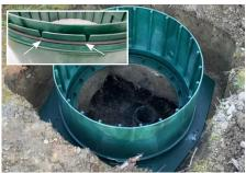
Add your riser to the adapter ring making sure to add the gasket around the face of the riser first - see *inset picture above*. Then use the hex head screws (supplied) to screw the riser into place.
