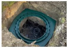
Clear enough space around your access hole to accommodate the adapter ring. Clean the surface of the concrete. Add the bitumen sealant around the base of the adapter ring. then fix the ring to the concrete with anchor bolts (not supplied).
