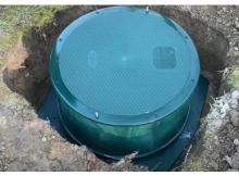
Add your cover when at finished ground level. Secure in place with the cover screws supplied. (A pedestrian dome cover is supplied as standard with integrated handles.)
