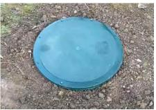
Backfill evenly around the risers up to the cover and the project is complete.
