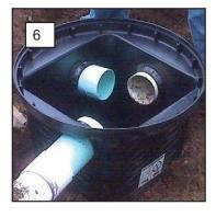
You are now ready to insert the correct size pipe by pushing it through the flexible watertight D-Box seal.
