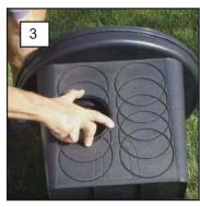
Check to make sure you have completely tightened the nut and that the seal is not loose on the D-Box.
